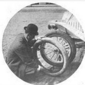
Fig. 1—First operation in adjusting Jenkins Emergency Wheel
