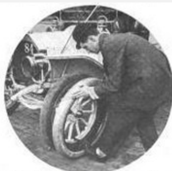
Fig. 2—Second operation, fitting emergency wheel in place
